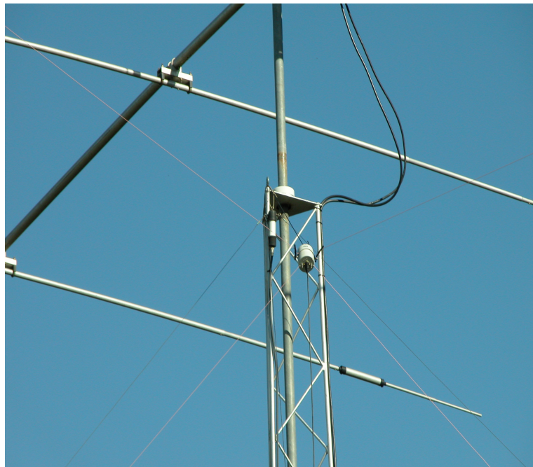
Illustration 5: Final Installation of Antenna
